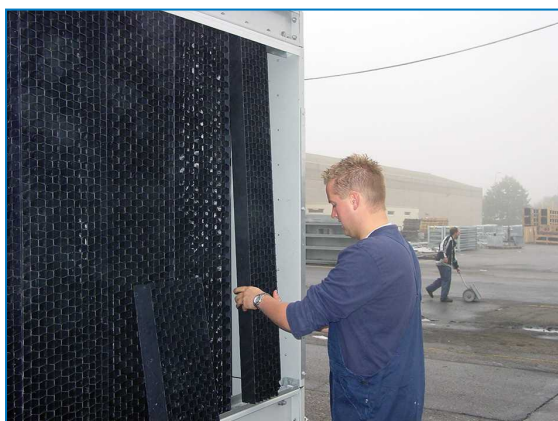
Remove combined inlet shields
