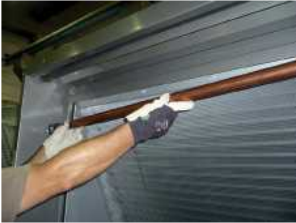
Remove copper waterfeed pipe
