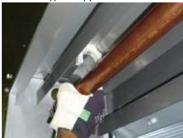
Release copper collector from plastic holders
