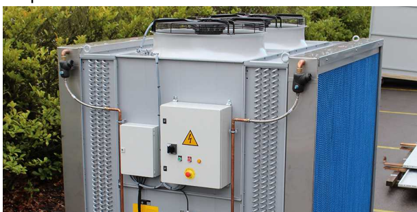
Waterfeed assembly connected to city water connection with flexible pipe
