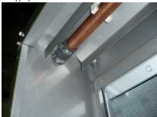
Flexible sleeve connection
