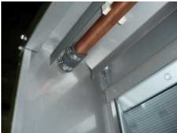
Flexible sleeve connection with sleeve clamps
