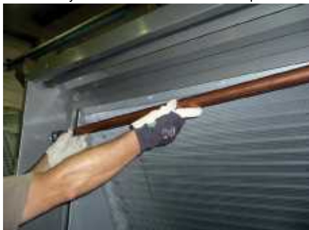
Remove copper waterfeed pipe
