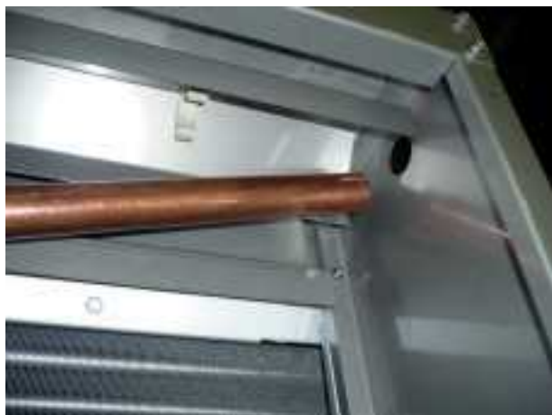
Installation of copper waterfeed pipe
