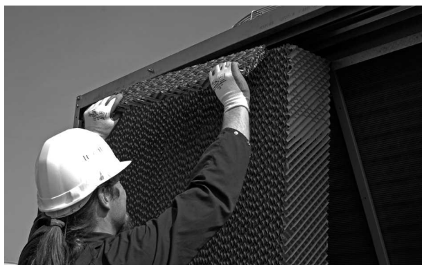
Removal water distribution pads
