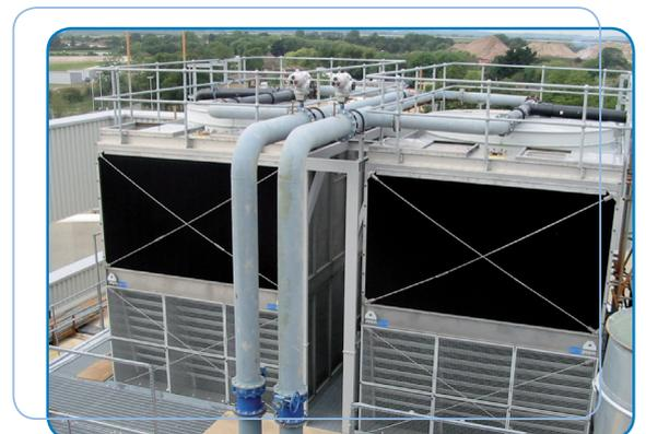
Combined Inlet Shields retrofitted to the top half of BAC S3000 cooling towers with old style louvres at the bottom
